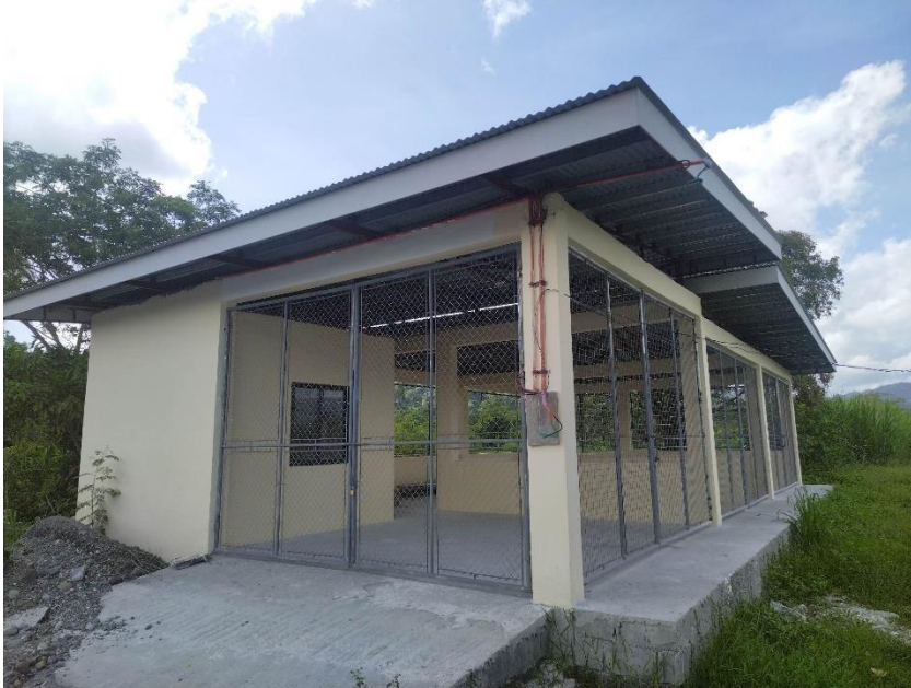
Figure shows the current Materials Recovery Facility of the Mindoro State University Victoria (main) campus.
